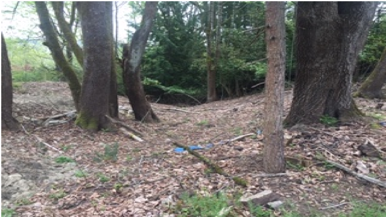
Photo 2: Looking east toward the southeast at the head of small gully that runs along the south side of the property.
